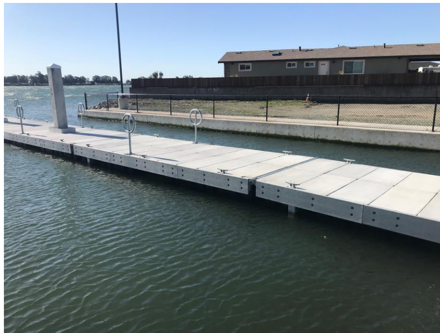
Pile-guided boarding float with retaining wall in the background
