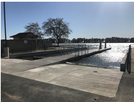
Two-lane boat ramp, pile-guided boarding float, security lighting & retaining wall
